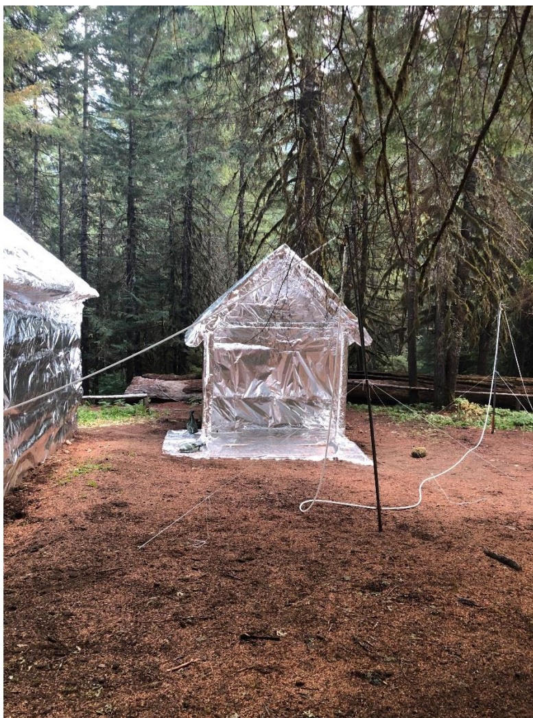
Wrapped Structures Bagby Hot Springs during the Bull Complex, Mt. Hood NF Photo by Scott Weishaar
