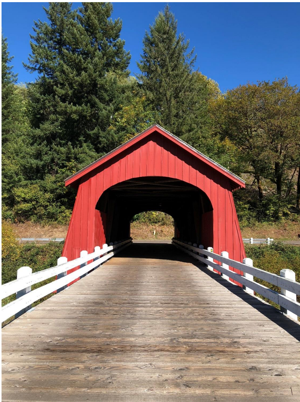
Fisher Covered Bridge – Central Coast Range of Oregon
