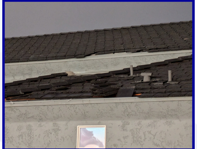
Roof Shingles blown off a house Photo by Josh Carstens
