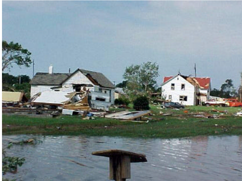
Damage in the town of Deshler from the F2 tornado that moved through the town. Photo by S. Kisner, GID WCM
