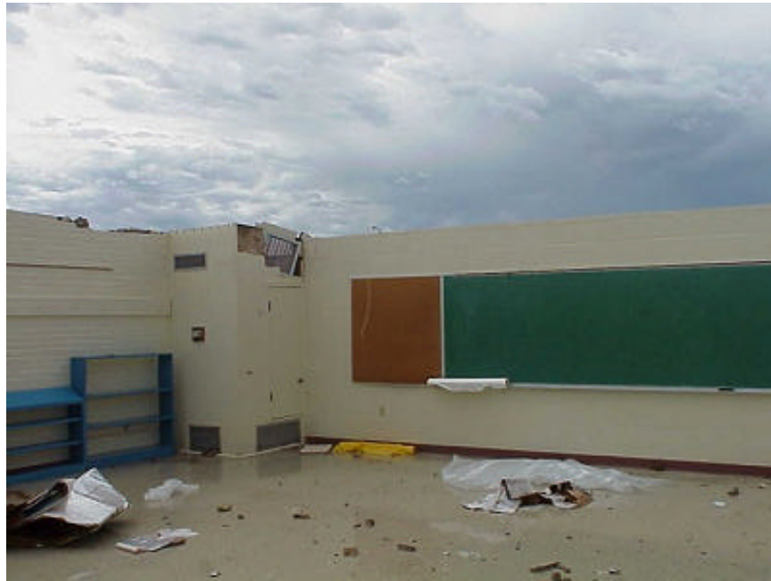
In the picture: Damaging straight-line winds removed part of the roof from an elementary school in Dumas (Desha County) on 06/11/2003.
