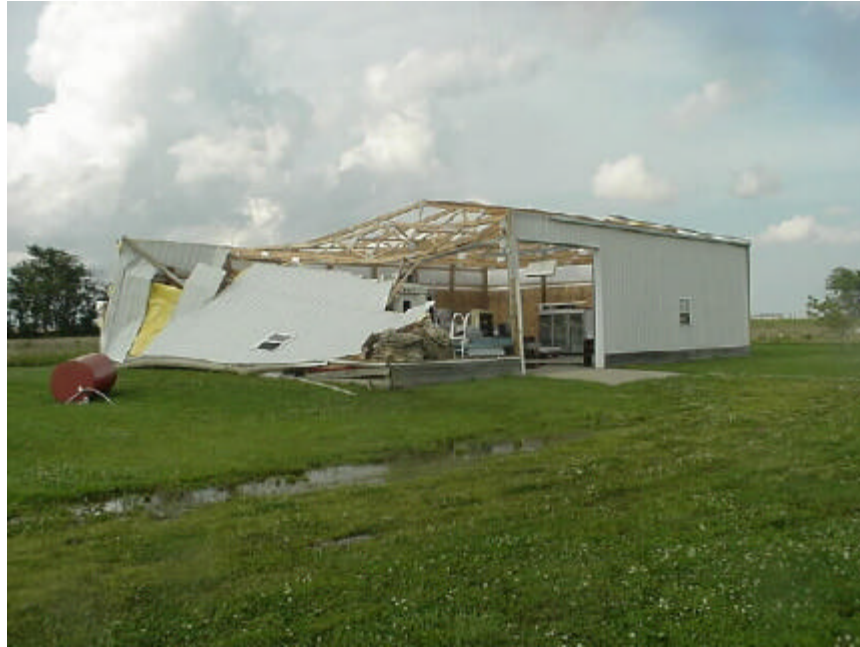
Barn/machine shed damaged near Plum Hill in Washington County, IL..
