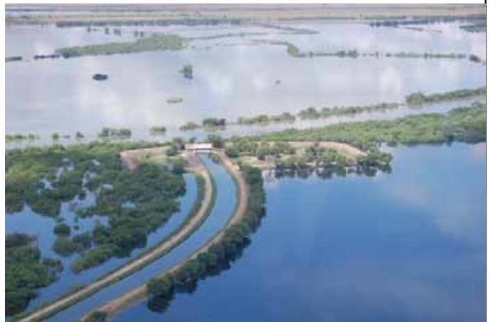
Flooding was severe in deep south Texas.
