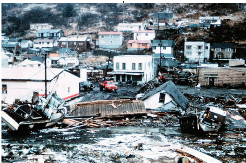
Tsunami damage at Kodiak, AK, after the 1964 Great Alaska Earthquake and Tsunamis.
