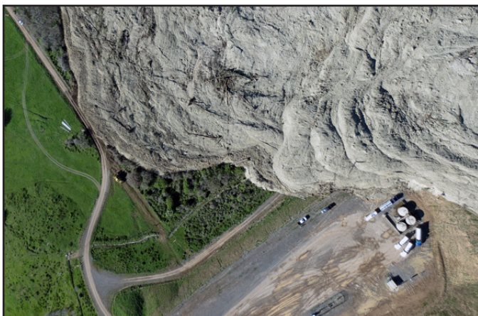
The toe of the landslide impinged on farmland and gas wells. Photo by Mesa County, CO, staff.
