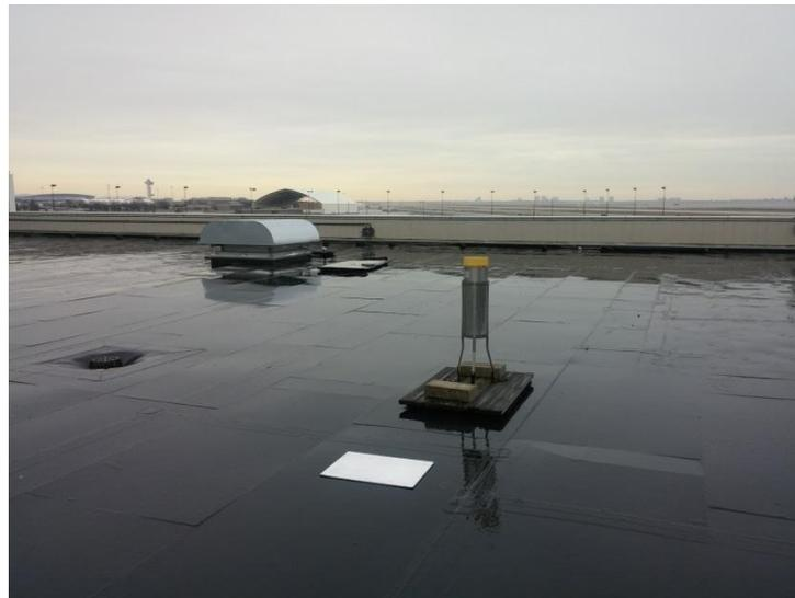
The primary area used for official snow measurements at JFK International Airport denoted by the white SMB in the photo. This is a view looking southeast. An 8-inch standard rain gauge is also located on the roof as a back-up to the ASOS at JFK.
