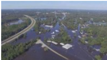
Aerial view of flooding in Princeville. Photo taken by NCDOT via WNCN.
