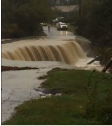
Road washed out on Greenock Avenue in Fayetteville. Photo taken by Fayetteville Police via WNCN.
