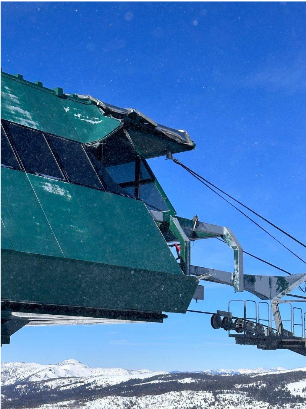
Figure 5. Wind damage to Chair 6 at Kirkwood Mountain Resort. Photo courtesy of Kirkwood Mountain Operations .
