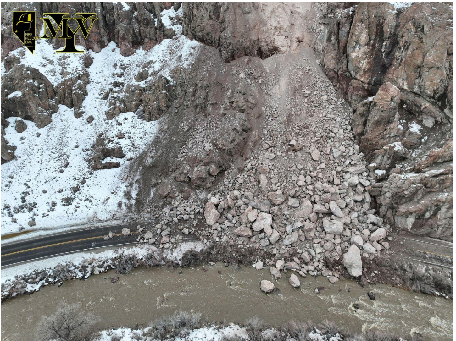
Figure 4. Wilson Canyon Rockslide over SR-208. Road closed for clean-up and repair on January 10th, still closed as of February 3rd. Photo credit: Yerington Mason Fire Protection District.
