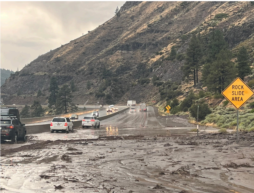
Photo 6, I-80 near Floriston, Wednesday 8/27 ~ 2:45pm, photo courtesy Caltrans District 3.
