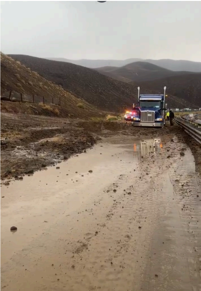
Photo 7, I-80 Westbound near Tracy Clark NV, Wednesday 8/27 ~ 4:30PM, photo courtesy NDOT.
