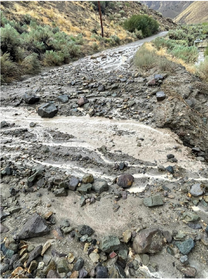
Photo 2: August 25th, Six Mile Canyon Road, Photo courtesy of Lyon County.
