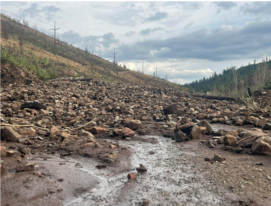
Photo 8: One of several debris flows impacting rural roads south of Loyalton CA. within the 2024 Bear fire burn perimeter. This is Smithneck Road after heavy rain on Wednesday 8/27. Photo courtesy of Sierra County Public Works.
