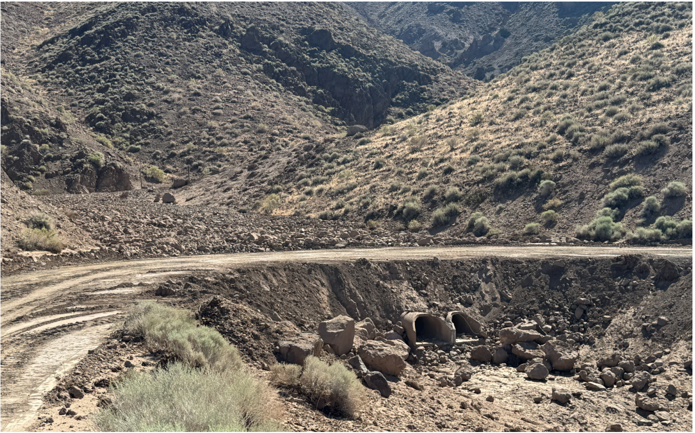
Photo 2. Debris flow material retained above road fill above Hidden Valley Neighborhood. Photo courtesy of Scott McCoy UNR
