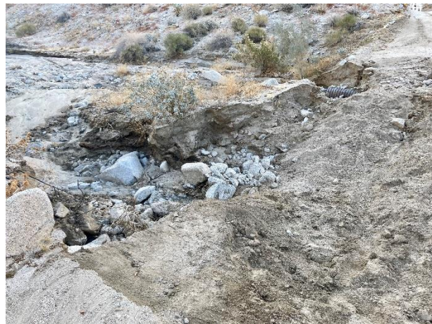
Intense rain ripped through Canebrake, washing out this creek crossing on 22 December (Natalie Spandau).
