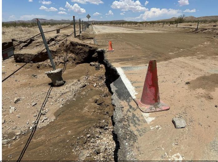
The damaging results of a flash flood near El Mirage after thunderstorms on 20 and 21 May (above, Alex Tardy).
