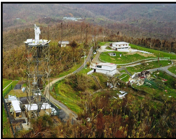
TJUA NEXRAD at Cayey, PR destroyed by Maria.
