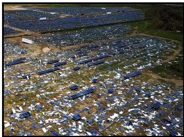
Major damage to the solar panel farm in Humacao, PR
