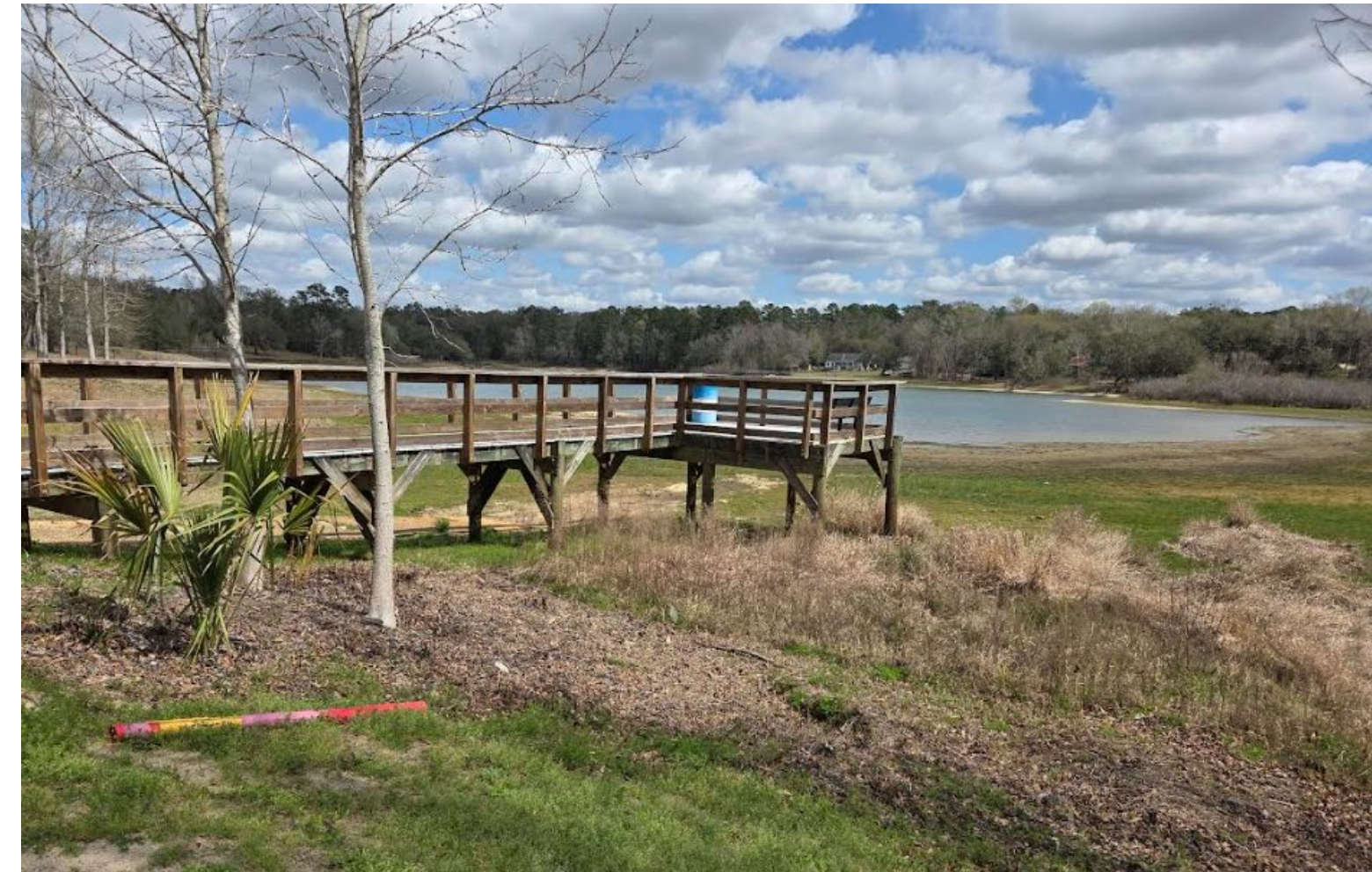
Courtesy Washington County EMA: Blue Lake in Chipley. Water is normally under the decking very near the mulching just to the right of the tree.
