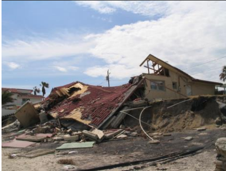
Major Dune Erosion: Undermines vulnerable Coastal structures
