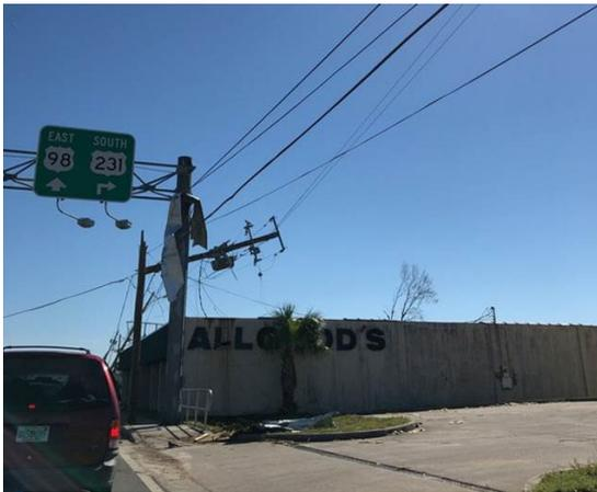
**Figure 51:** Damaged electric pole near West 15<sup>th</sup> St., Panama City (Latitude: 30.175136, Longitude: -85.663061).
