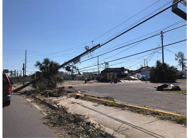
**Figure 50:** Damaged electric pole near West 15<sup>th</sup> St., Panama City (Latitude: 30.175136, Longitude: -85.663061).
