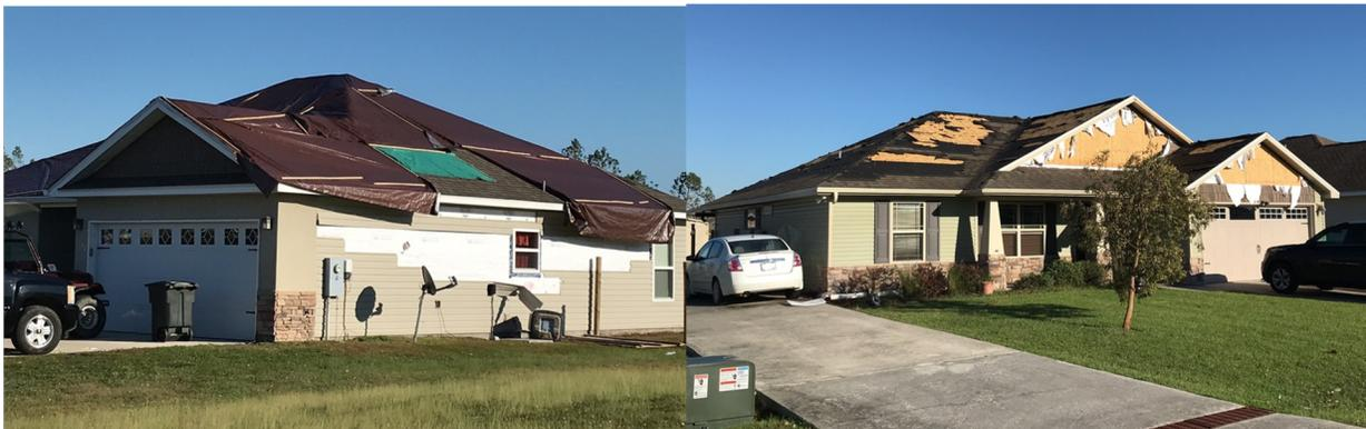
**Figure 10:** Damage to roof cover and building wall envelope observed in Southport
