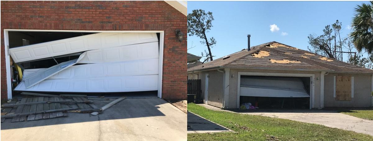
**Figure 21:** Garage door failures in residential homes in Cedar's Crossing.
