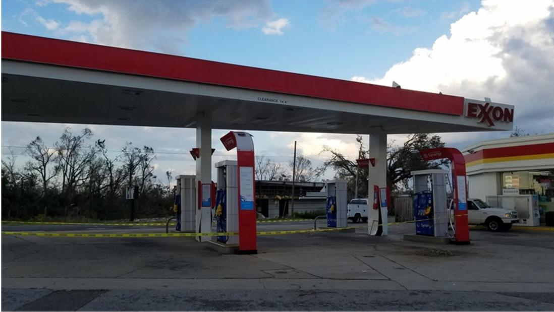
**Figure 44:** Exxon station sustaining column and roof damage at US 90 in Marianna.
