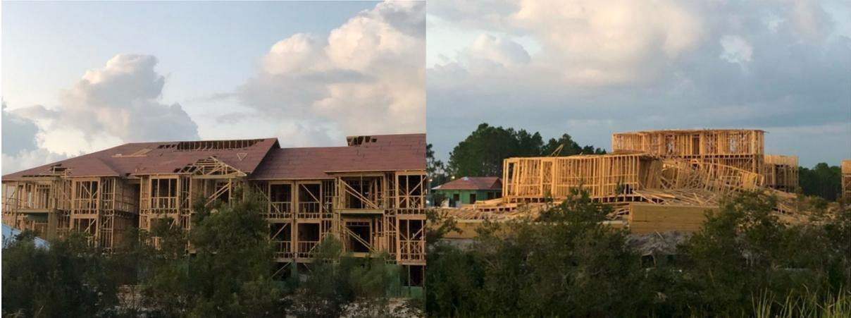
**Figure 13:** Construction sites in Panama City Beach sustaining moderate wind damage.
