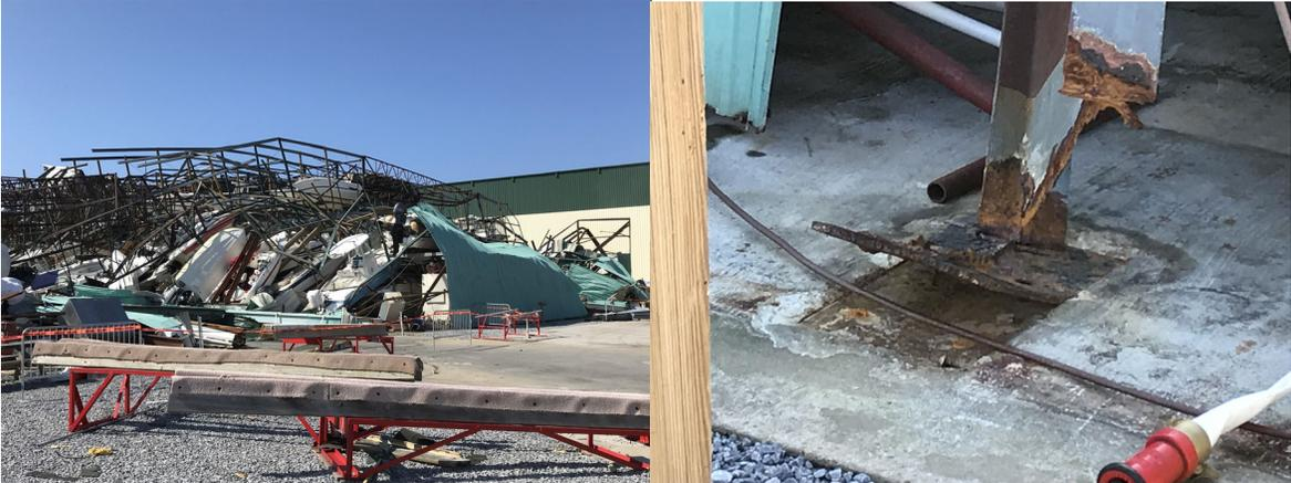
**Figure 14:** Collapse of a storage building (left) with corrosion and material loss in columns and baseplates (right).
