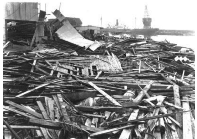
Destruction at the Southern Steamship Co. and Gulf Terminals, Tampa.*
