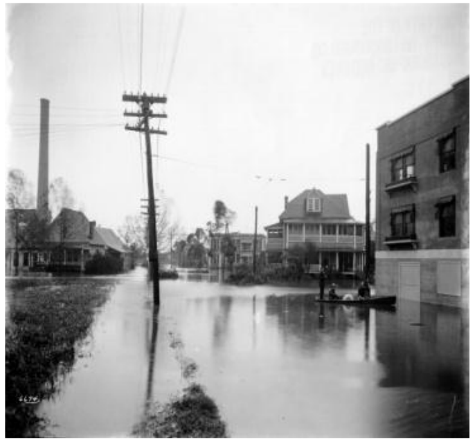
The storm surge brought extensive urban flooding as shown here at the intersection of Parker and Eagle streets, Tampa.*
