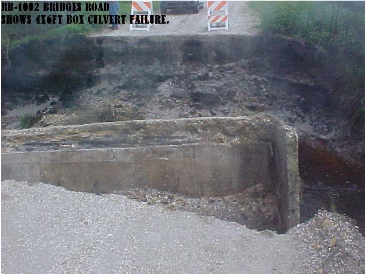
Hardee County Road Washout - Photograph from Bill Muhlfeld, Hardee County Director of Emergency Management.
