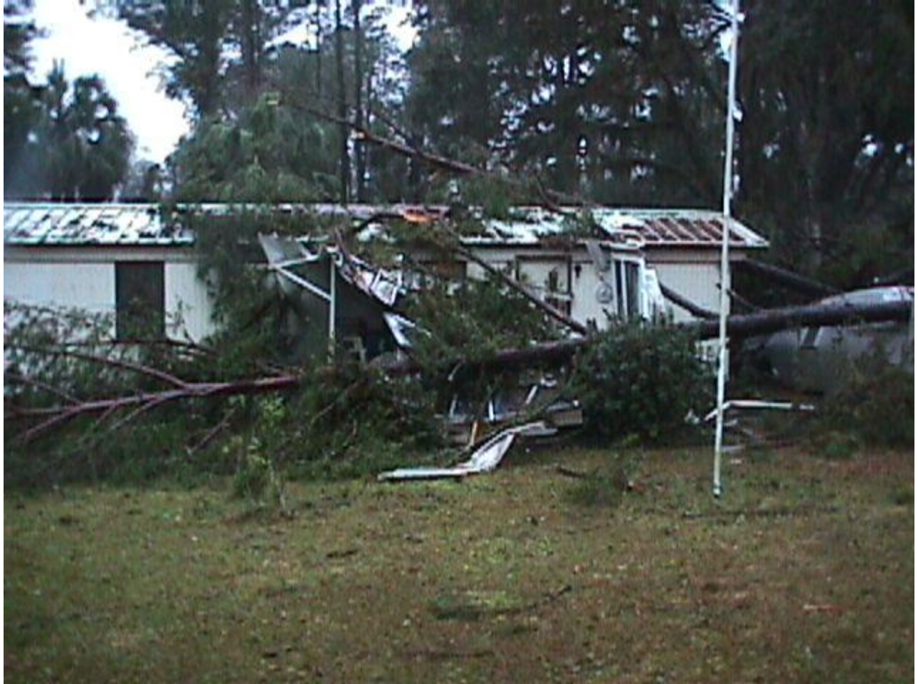
Damage to a home in the Derosa area, near Lake Rousseau, in extreme northern Citrus County.
