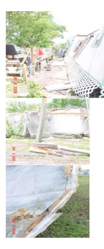
Un-anchored single-wide mobile home pushed 4 to 5 feet from original position. Mobile home roof was blown off and walls partially collapsed. Notice the almost intact trees to the west of the home. Several small 4 inch diameter branches were broken; however, trees remained mostly intact.
