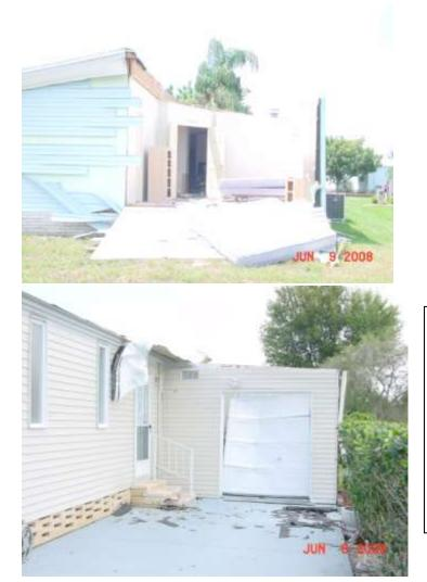
Double-wide mobile home with complete structural failure of outer wall and roof section. Wall joints were screwed together 2X4 sections with 2X4 pieces split vertically. Wood was not rotted.
