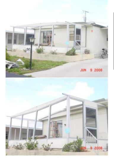
Double-wide mobile home with roof damage. Screened porch (lanai) severely damaged with roof missing as well as outer walls. Mobile home aluminum roof shredded in places.
