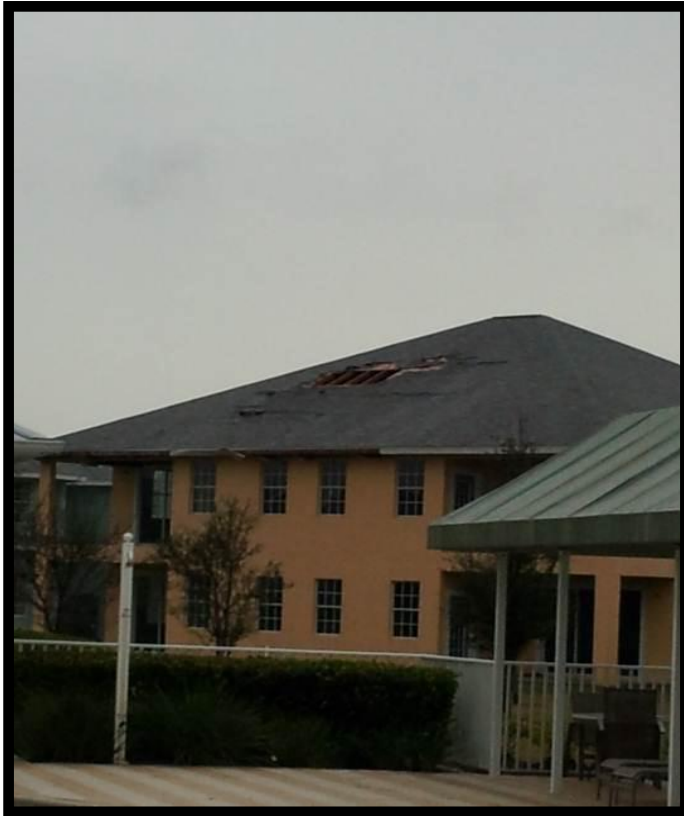
Tornado Damage at Point 1. Courtesy of Charlotte Co. EM
