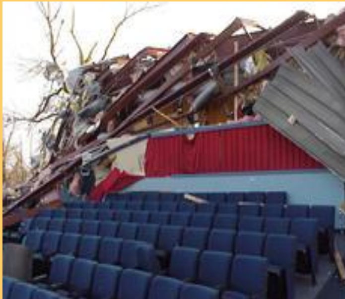
Cinema Damage from F4 Tornado in Van Wert, Ohio. Advanced warning systems used by the theater manager averted potentially dozens of casualties.
