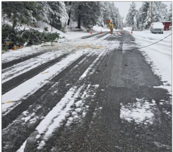
Power line damage in Jefferson County. Image Credit : Jefferson County Volunteer Fire
