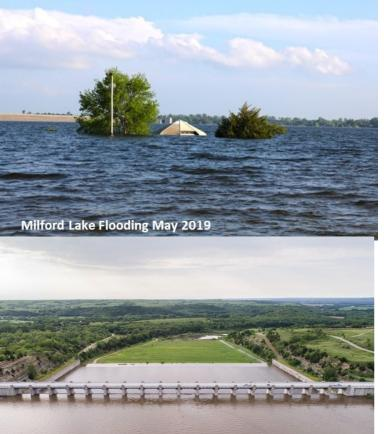
Water held back by spillway gates May 29 2019 at Tuttle Creek Dam. Lake elevation was ½ foot away from the top of emergency spillway gates. Photo by Ray Martinez
