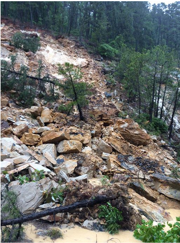
Fig. 52. ODOT: This rock slide impacted the safety of the road bed of US-259 about five miles south of SH-63 in LeFlore County on May 25, 2015. http://www.ok.gov/odot/Flooding2015.html
