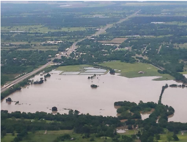
Fig. 33. Poteau River 5/12/2015 2:30pm CDT (PANO2 42.11') "This is the water treatment facility mentioned in the impact statements. The water was less than a foot from going over the berms. (Michael Davidson, Image)" "The pond to the north is pond 1 raw sewage. The pond in the right corner is pond 4. It's the one that is pumped to the river, but in this case, the river almost came to it (David Fox, takes care of the pumps there)."
