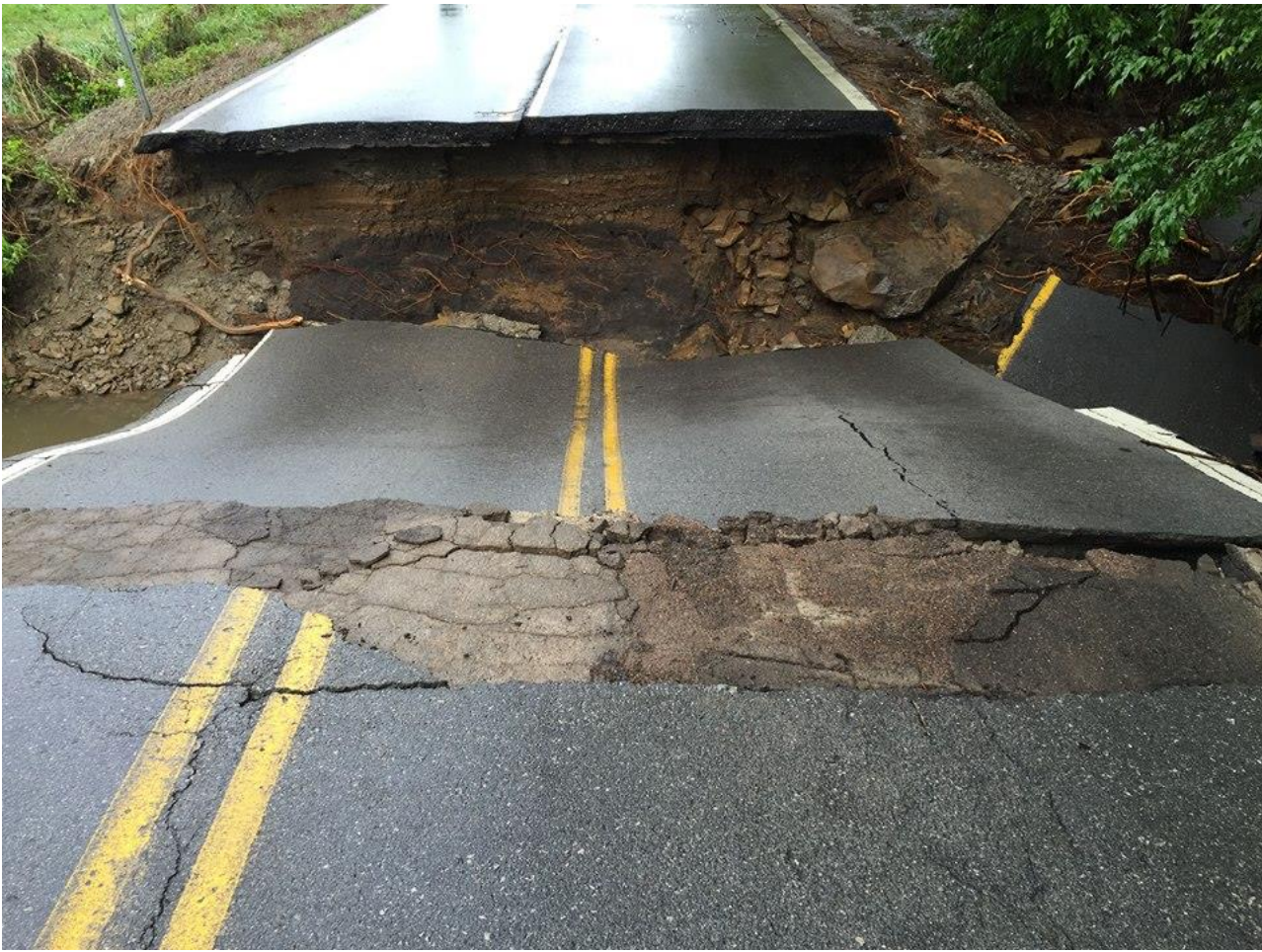
Fig. 63. Part of 61st Street between 209th and 193rd in Broken Arrow, OK was washed out by flood water. Fox23 5/24/2015
