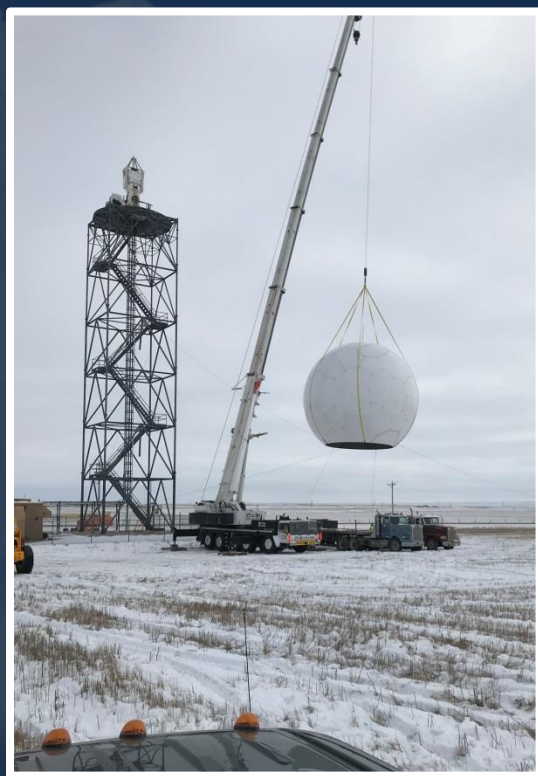
The dome comes off! Our radar dome was removed, and the antenna pedestal was replaced, on the morning of December 6th.
