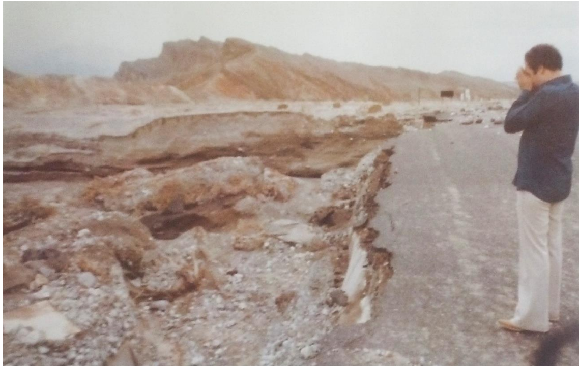
Damage caused by flash flooding along the Furnace Creek Wash in August 1984. Photo Courtesy: Furnace Creek Inn.
