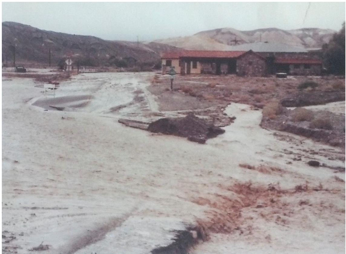
Flash flooding on the Furnace Creek Wash in August 1984 damaged roads. Photo Courtesy: Furnace Creek Inn.
