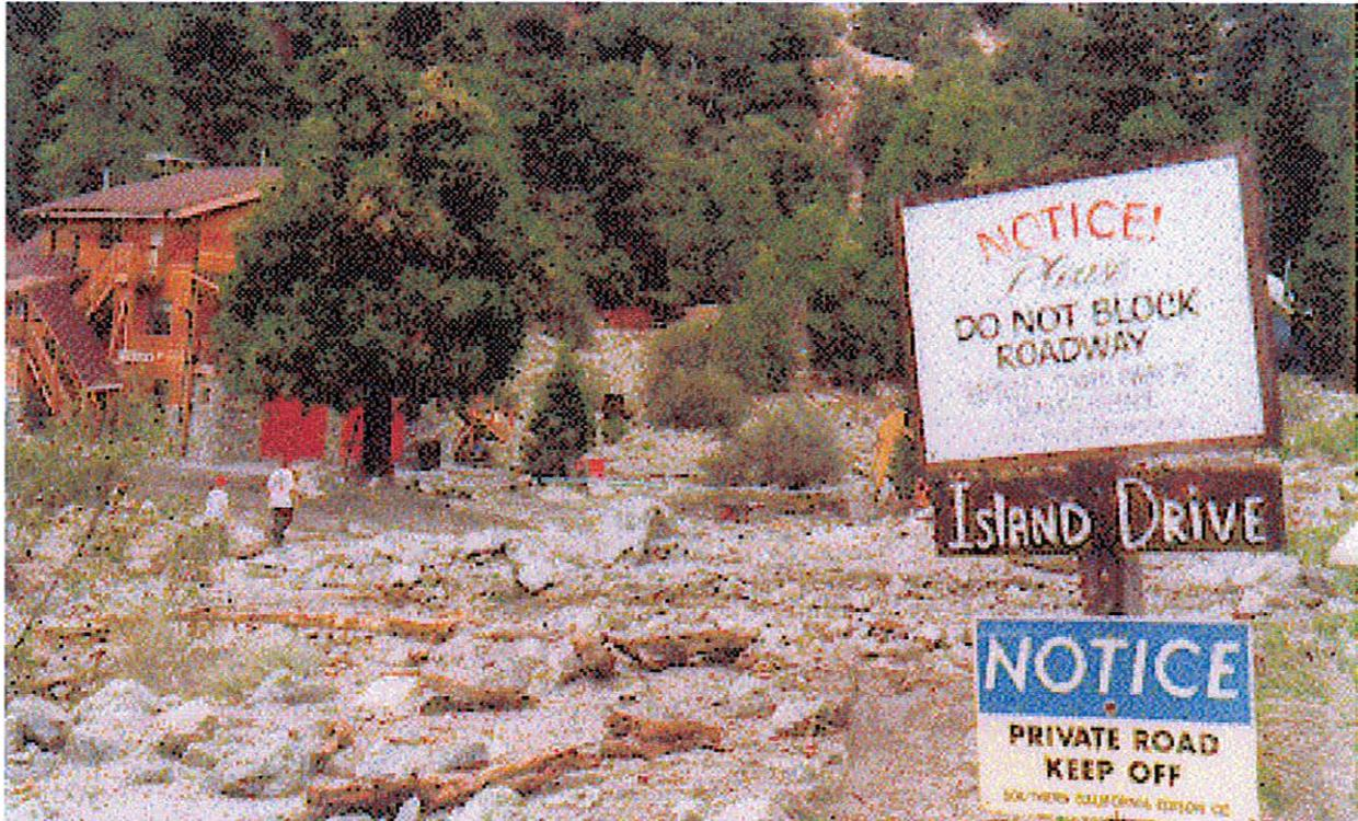
**Fig. 4. Roadway covered by large boulders.**
