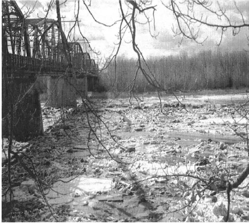
Figure 9. Photograph of the Yellowstone River on March 20, looking west along the Bell St. bridge (at left of photograph) in Glendive.
