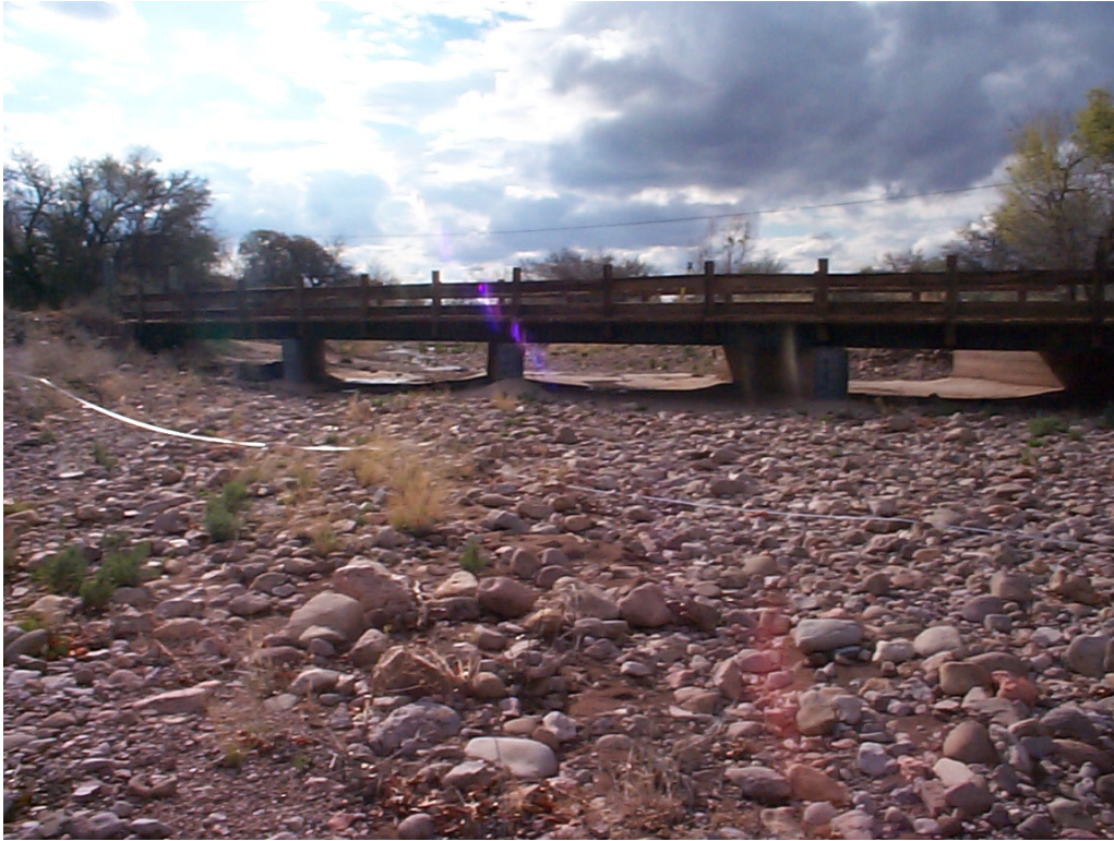
Figure 18: Cross section 6 looking downstream towards Rucker Bridge. Cobbles dominate channel bottom as well as banks.
