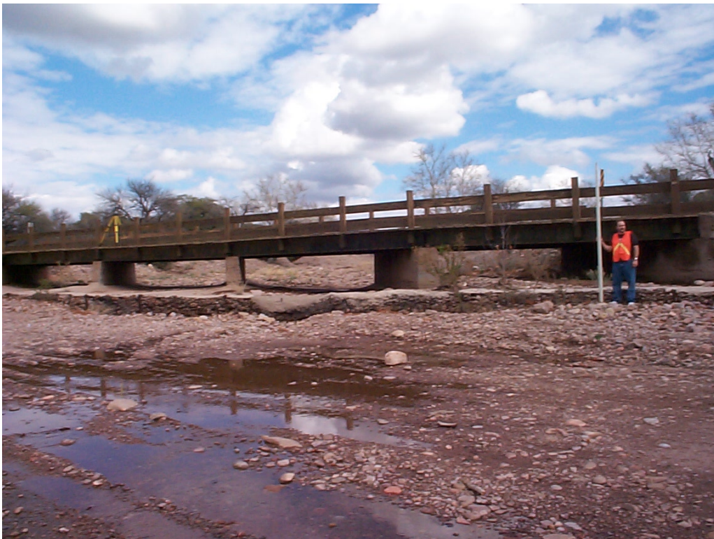
Figure 19: Rucker Bridge as seen from low water crossing just downstream of bridge. Yellow survey tripod seen on downstream-north side of bridge.
