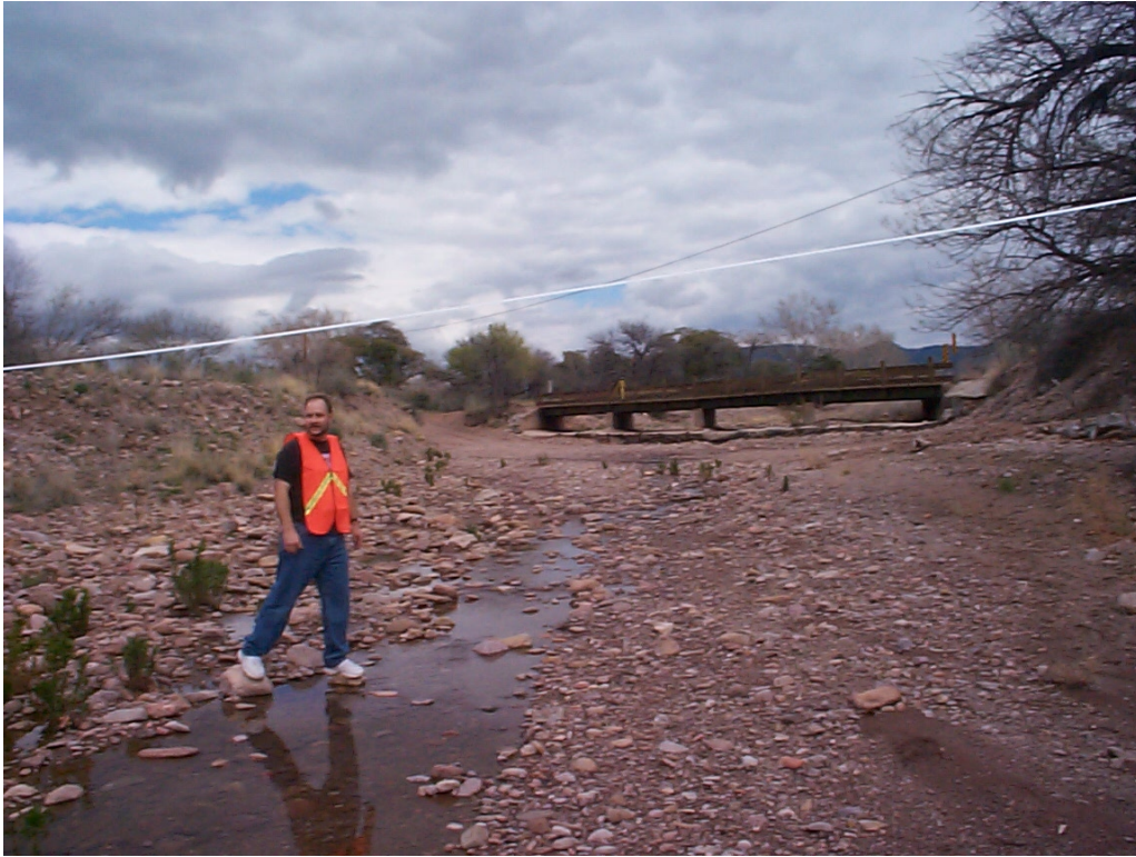
Figure 14: Cross section 2 looking upstream. Tape measure shows approximate position of cross section. Rucker Bridge and adjacent low water crossing seen in distance.
