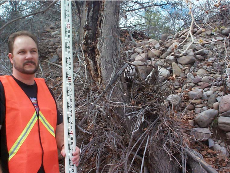
Figure 17: High water mark located at right bank of cross section 2. Debris, including a metal arrow bent by the flow, was discovered within.
