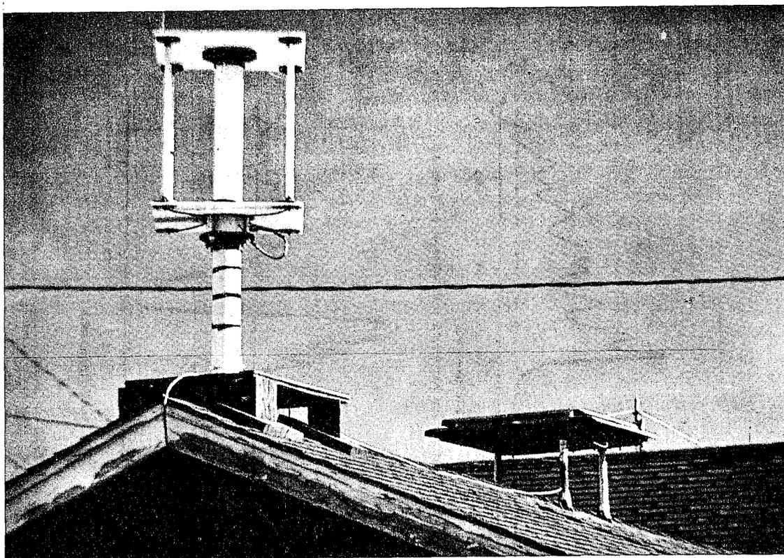
Figure 4. ALDS Antenna Array At Susanville, California.
