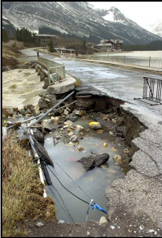
Figure 12. Bridge over Swiftcurrent Creek after water levels subsided. Water continued to fill the channel under the bridge at a near capacity rate. Damage here is on the approach to the bridge (courtesy National Park Service).
