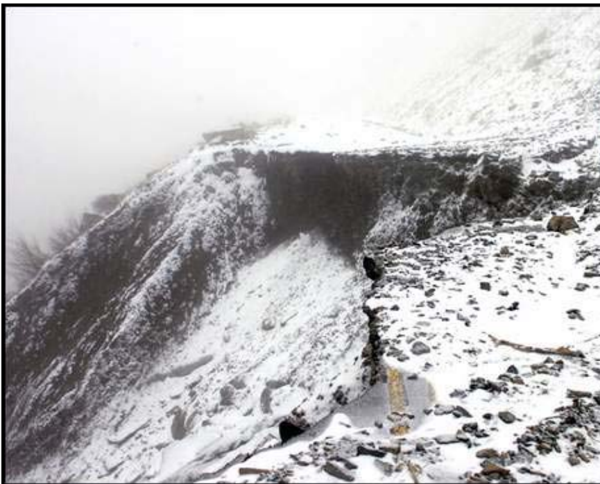
Figure 13. Going to the Sun Road in Glacier National Park washout on 7 November 2006. This is on the east side below the tunnel east of Logan Pass. Note the center line of the road in the picture (courtesy National Park Service).
