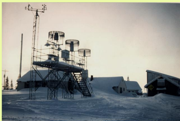
Figure 1 – View of Stampede Pass weather station in winter.
