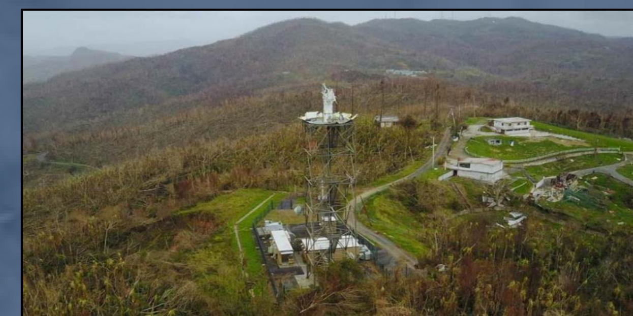
WSR-88D TJUA destroyed (NWS San Juan)
