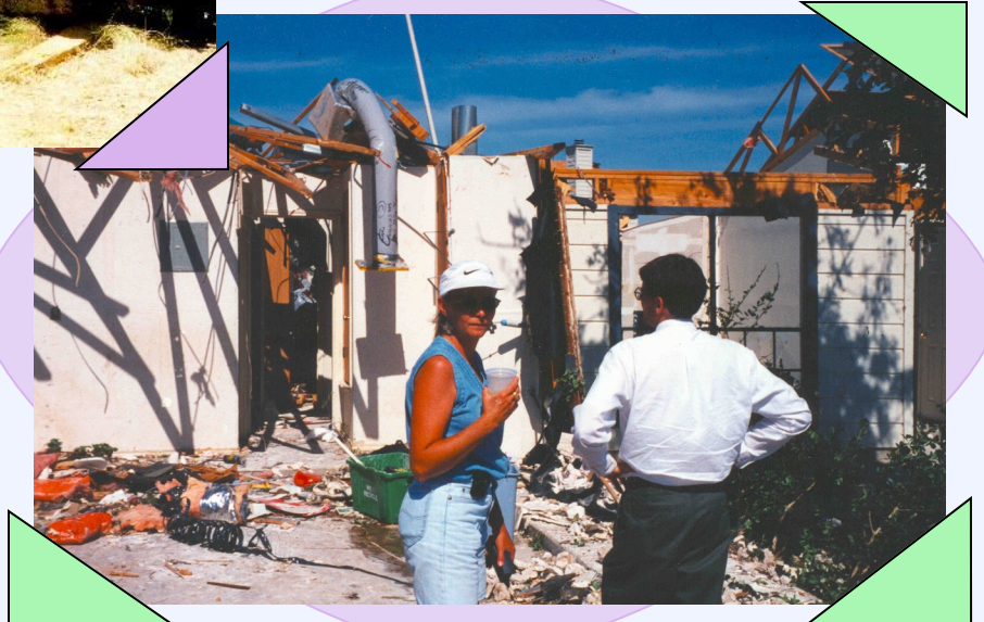
Figure 3. Home destroyed in Cedar Park by the F3 tornado. Several people took shelter in a utility closet, shown just to the left of the woman in the picture.
