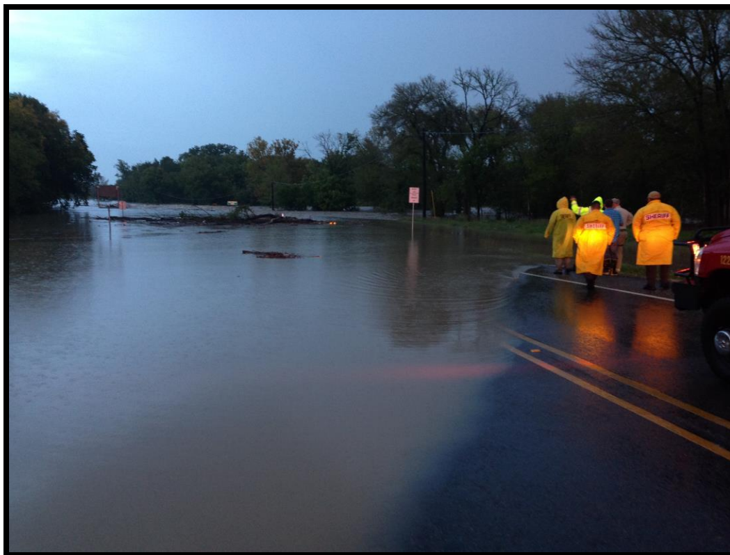
Figure 3. The San Marcos River flooding over FM 1979 near Martindale, TX, around 8:00 am October 31, 2013.
