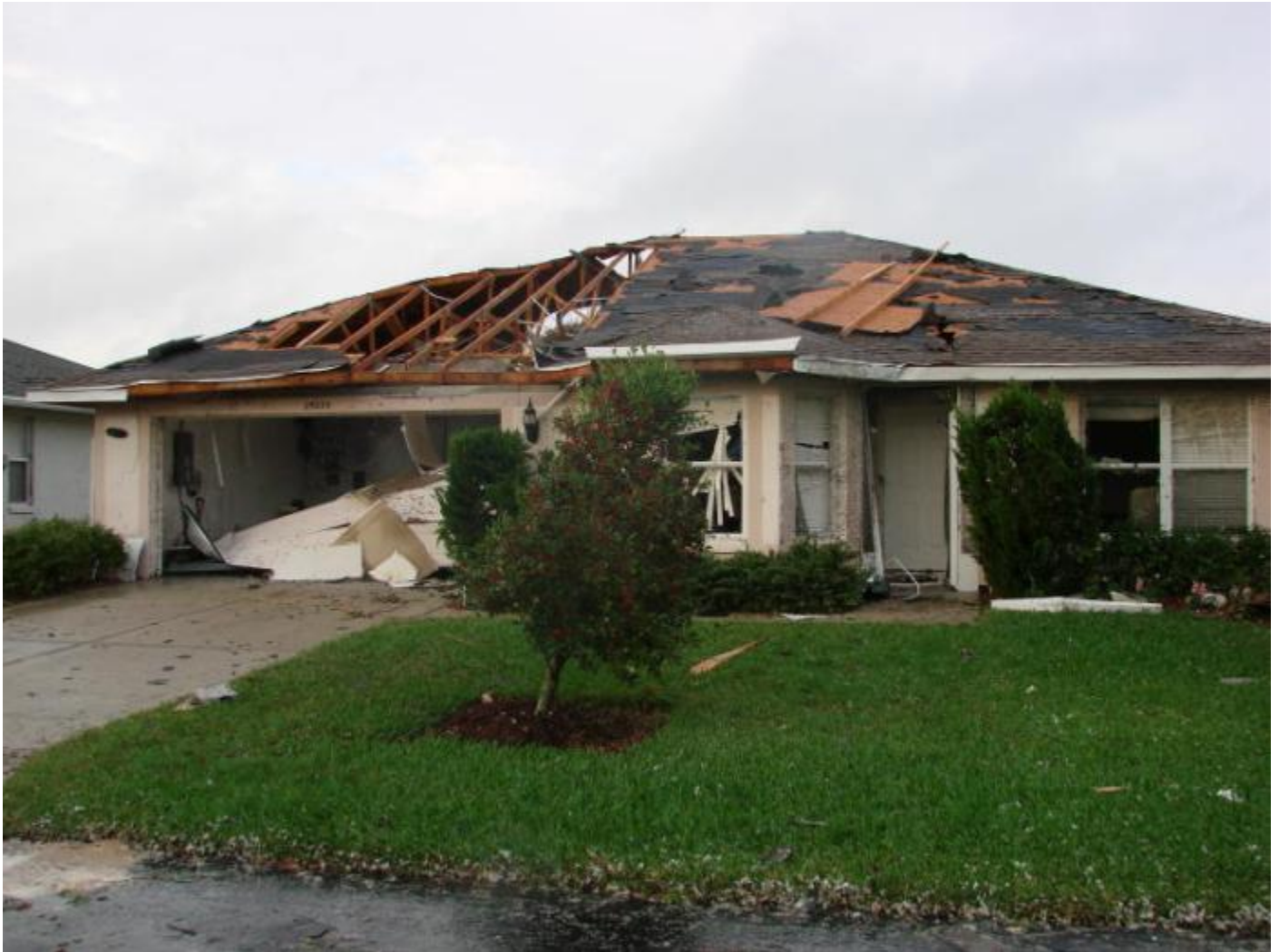
Photograph of F2 damage to home in the Tampa Bay Golf and Country Club
