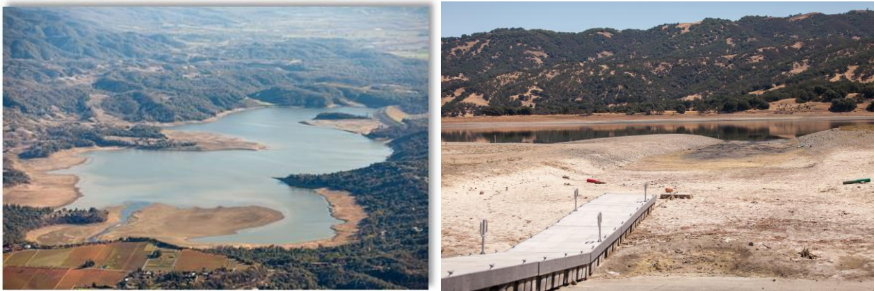
Lake Mendocino: Aerial view and plane view (courtesy SCWA)
